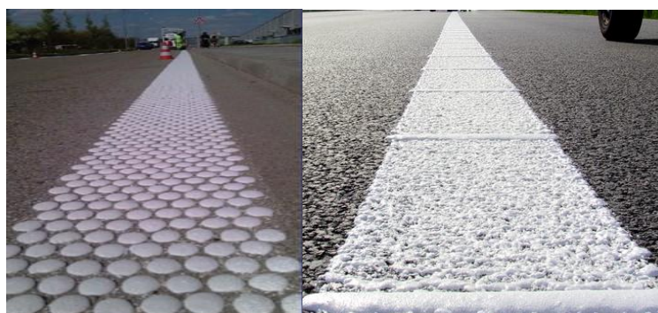
Figure 1 - Profiled road markings made by cold plastic
