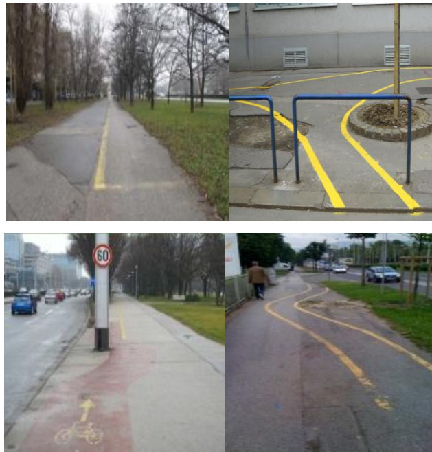
Figure 2 - Examples of improperly maintained (left) and executed (right) bicycle lines in the City of Zagreb
