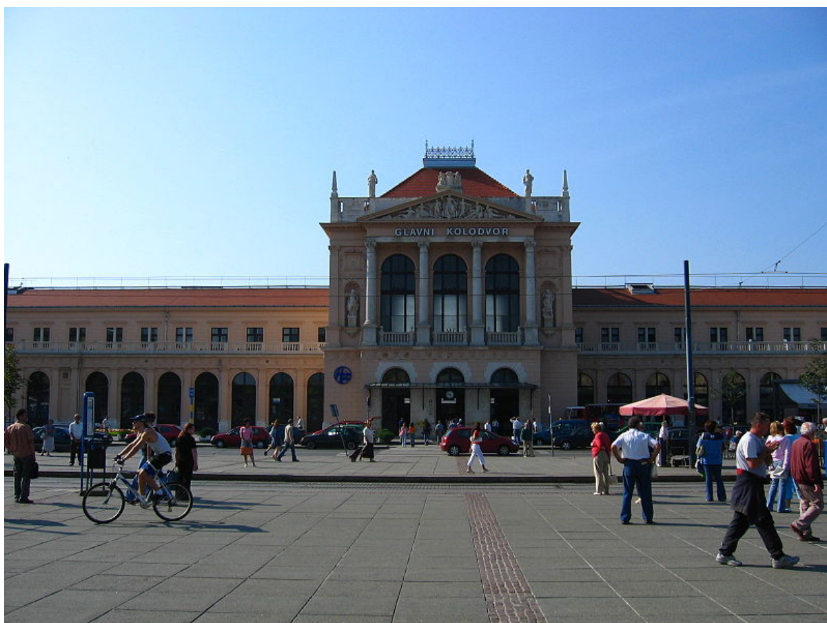
Figure 3 – Zagreb Central Station Building
